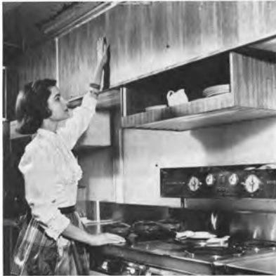
Wall-cabinet interiors behave like elevators, the cupboard shelves dropping down for use. It's done by a wave of the hand creating an electrical impulse which activates the switch that does the business
